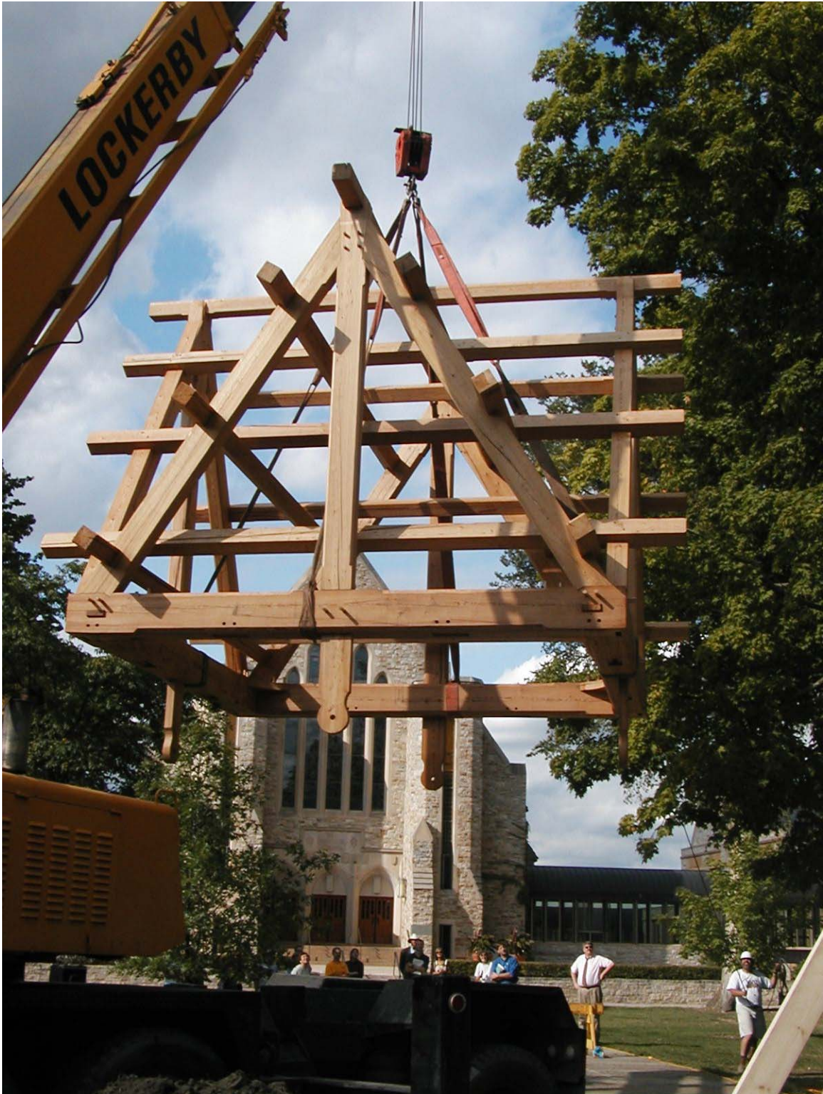
Figure 3. Assembly of the Memorial Chime Tower, 2003. Copyright 2003 by St. Gregory's College. Reprinted with permission.
